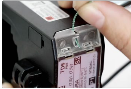
Once the terminal cover has been placed, the transformer sealed.
